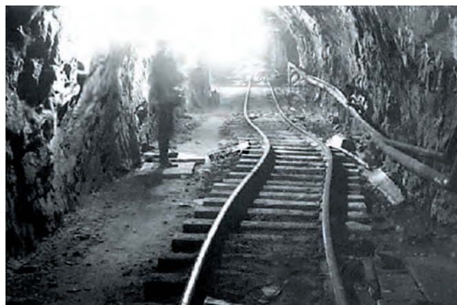
Fig. 8 Changes in the mine cross-sections as the result of dynamic manifestations of rock pressure
