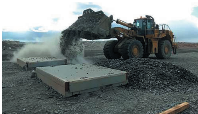
Fig. 1 Installation of the weighing platforms
